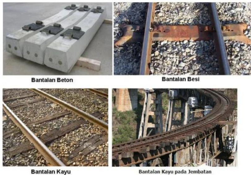
Figure 2. Different kinds of railroad bearing
